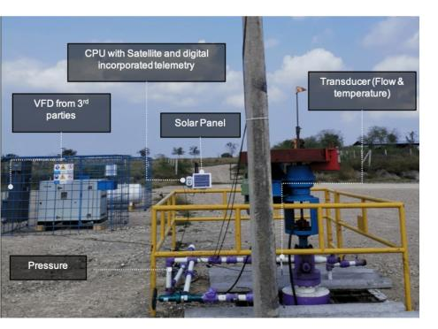
Flow, temperature, pressure and VFD's variables (RPM, torque, power, etc.)
